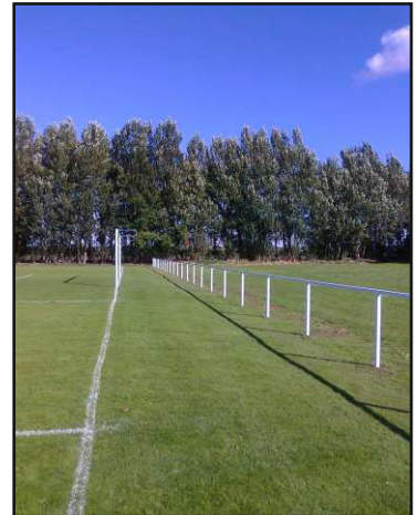
2.4m Rail with 1.5m socketed Post (0.5m underground) Thorne Colliery FC - Doncaster
